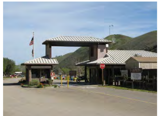
Carnegie SVRA entrance station
