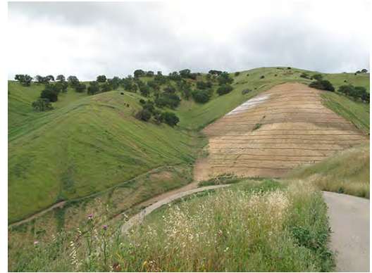
Wattles were placed on a hillside as a step toward rehabilitating the vegetation
