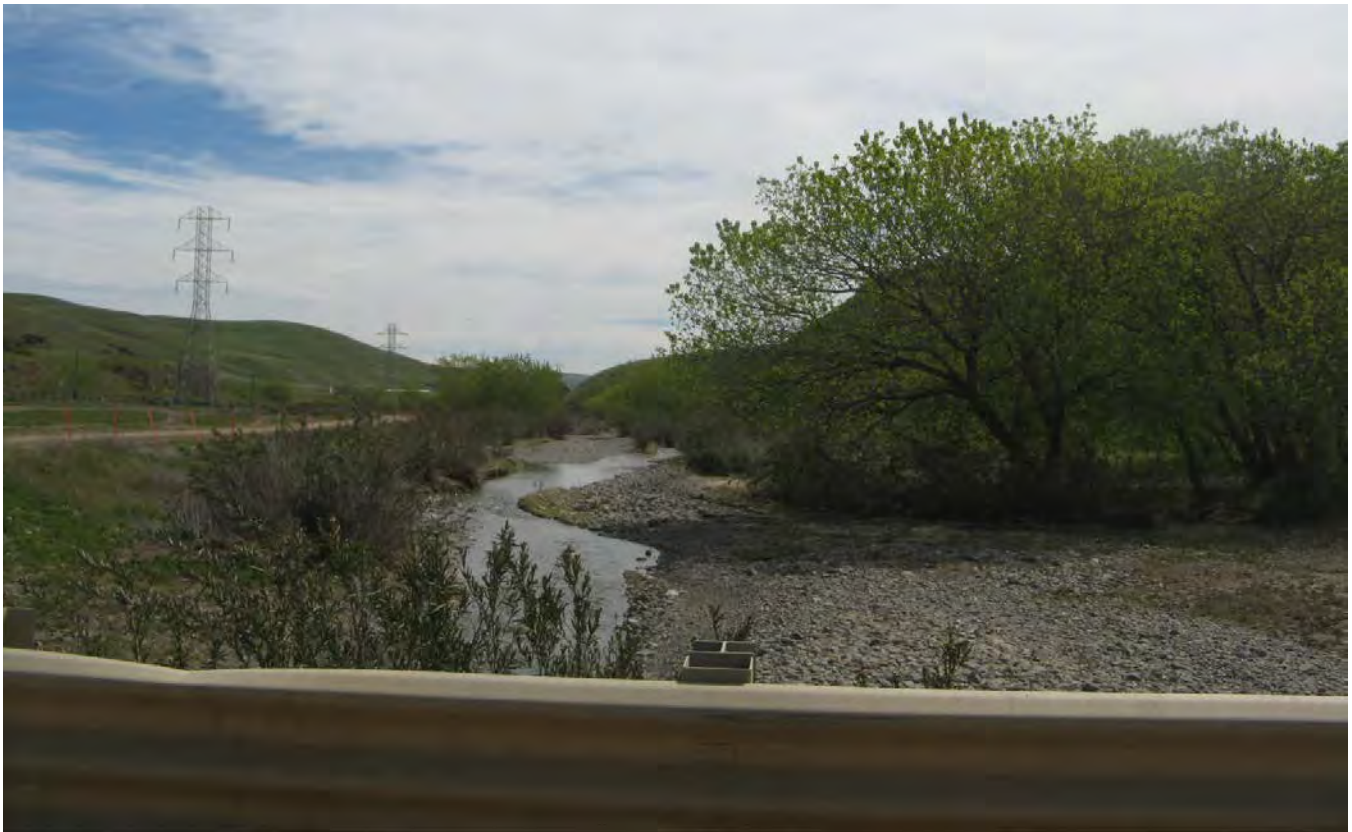
Viewpoint 3: View of Corral Hollow Creek facing east from the bridge at the Maintenance Yard. Note the power lines along Corral Hollow Road at left.
